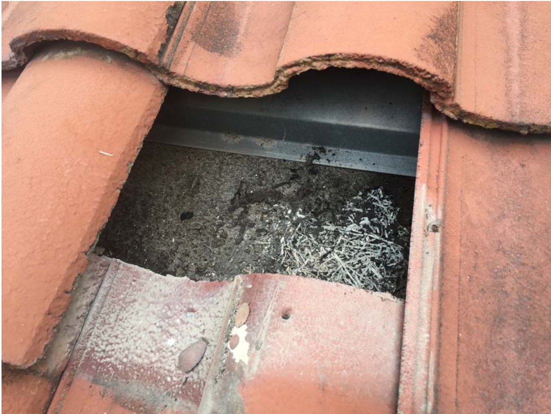
PHOTOGRAPH 5. THE COURTYARD TILE ROOFS ARE INSTALLED OVER CEMENTITIOUS WOOD FIBER (TECTUM) STRUCTURAL PANELS WITH AN ADHERED UNDERLAYMENT WITH GALVANIZED STEEL Z-FURRING CHANNELS.
