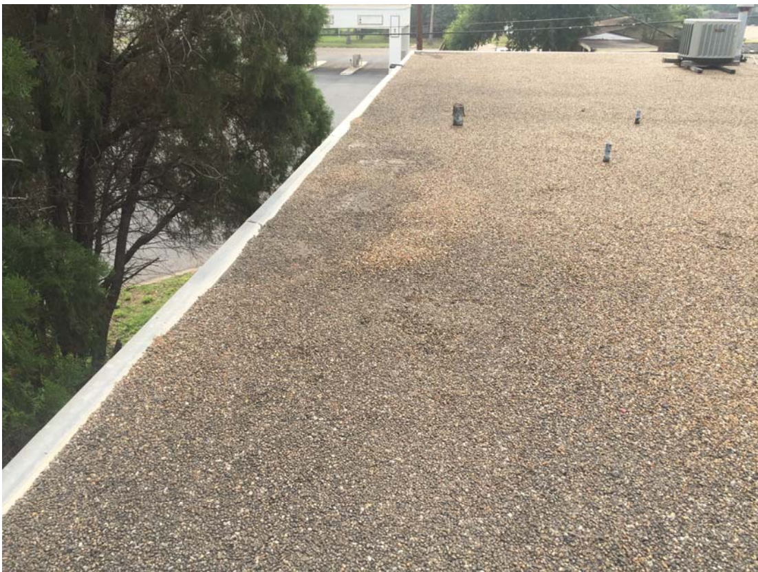
PHOTOGRAPH 20. SAME AS NOTED ABOVE.
