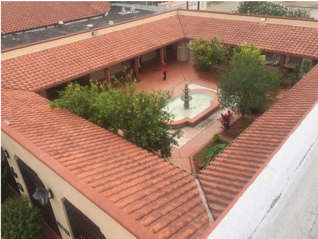
PHOTOGRAPH 4. OVERVIEW OF THE TILE ROOF COURTYARD (AREA 2) BELOW JUST TO THE NORTH SIDE. THE THEATER & A.V. (AREA 3) CAN BE SEEN IN THE BACKGROUND.
