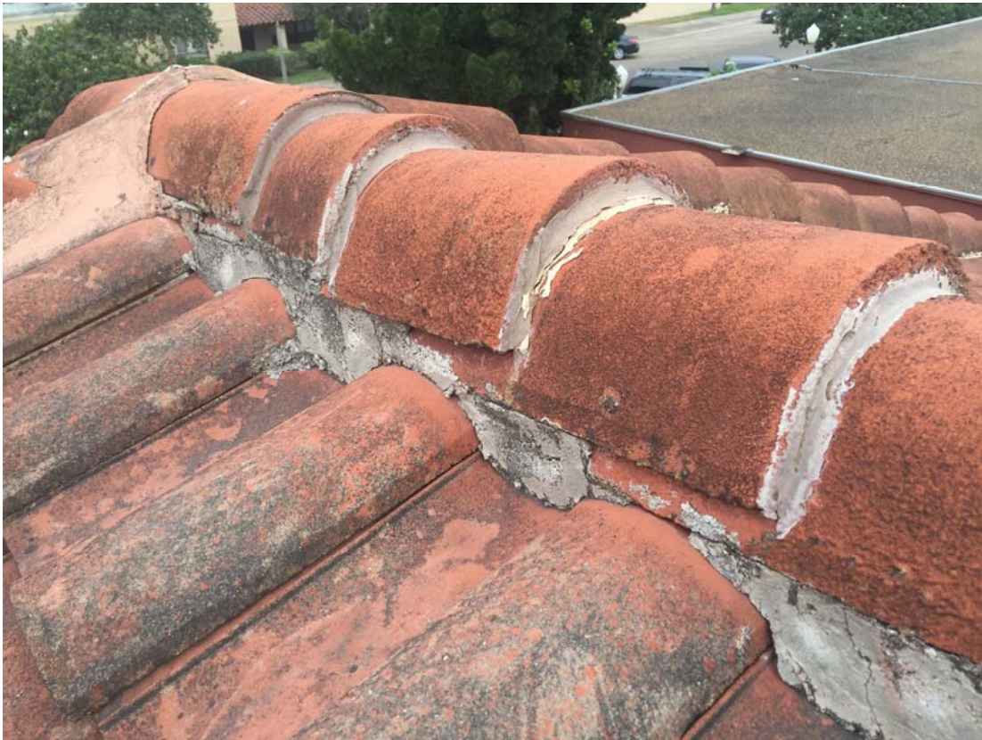
PHOTOGRAPH 15. SAME AS NOTED ABOVE.
