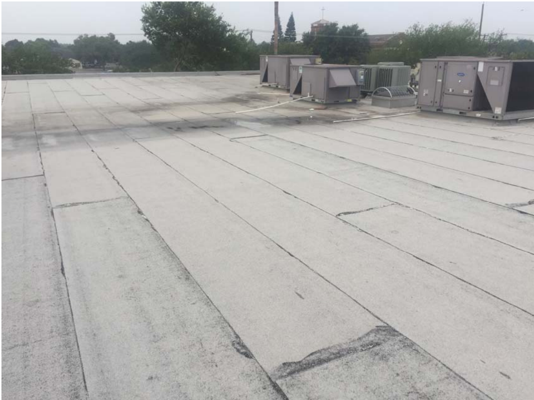
PHOTOGRAPH 2. ANOTHER VIEW OF SBS MODIFIED BITUMEN ROOFING SYSTEM OVER AREA 1.
