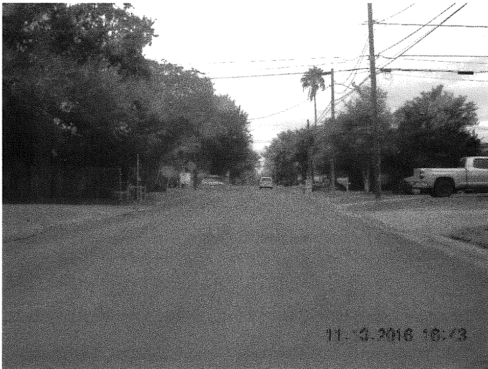
12) Picture taken facing west on 8 th street between Iowa Ave. and Tennessee Ave.
