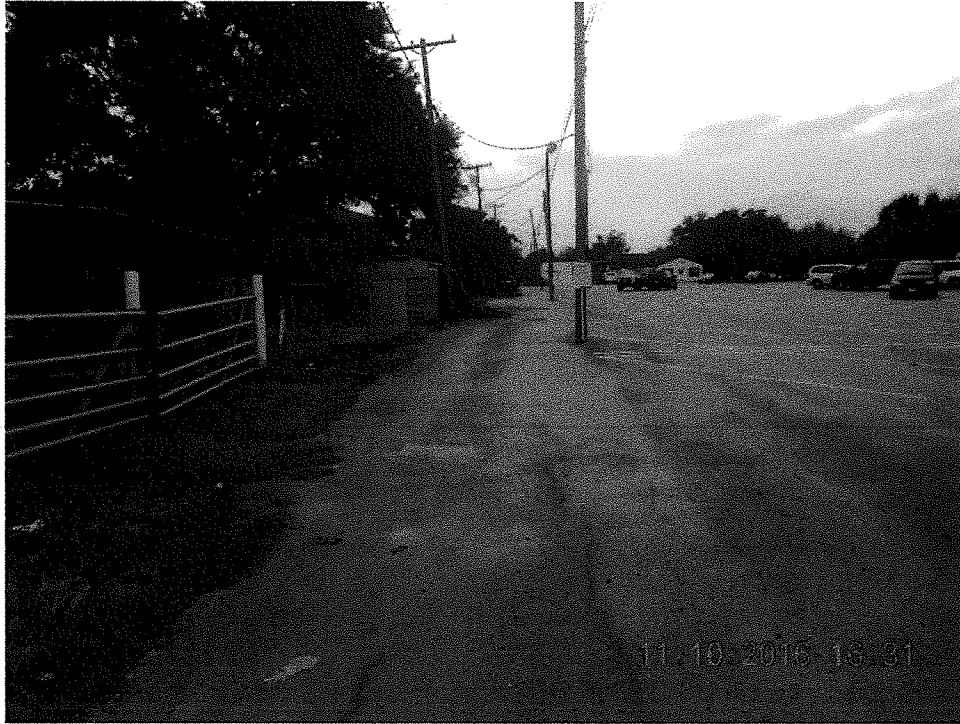
3) Picture taken facing south on alley of 6 th street between Kansas Ave and Illinois Ave.
