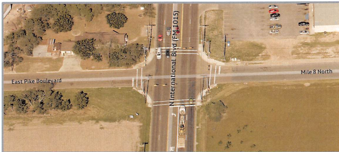
Figure 6 – International Boulevard & Pike Boulevard
