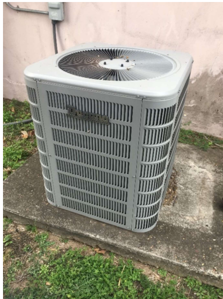
Figure 12: Replaced Split-System at Weslaco Tower Theatre (Outdoor)
