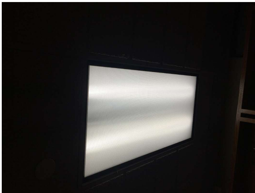
Figure 19: 2x4 LED Light Fixture at Public Library
