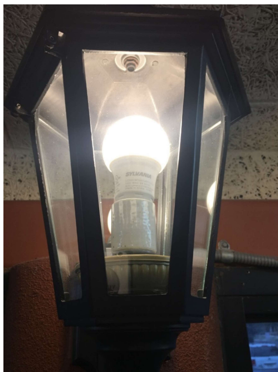
Figure 18: Screw-In LED Lamp at Public Library
