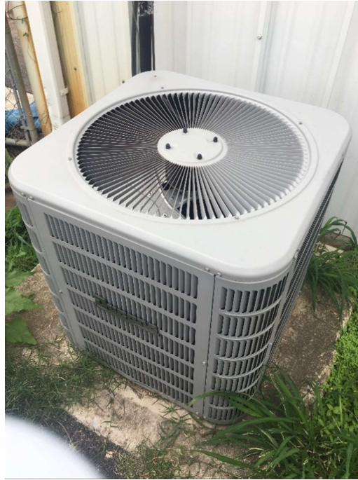
Figure 14: Replaced Split-System at PFA Building (Outdoor)
