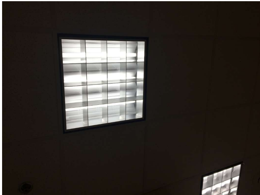
Figure 17: 2x2 LED Lighting Fixture
