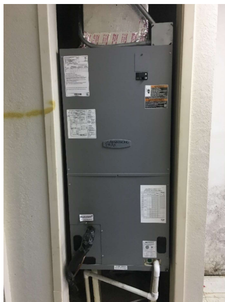
Figure 13: Replaced Split-System at Weslaco Tower Theatre (Indoor)
