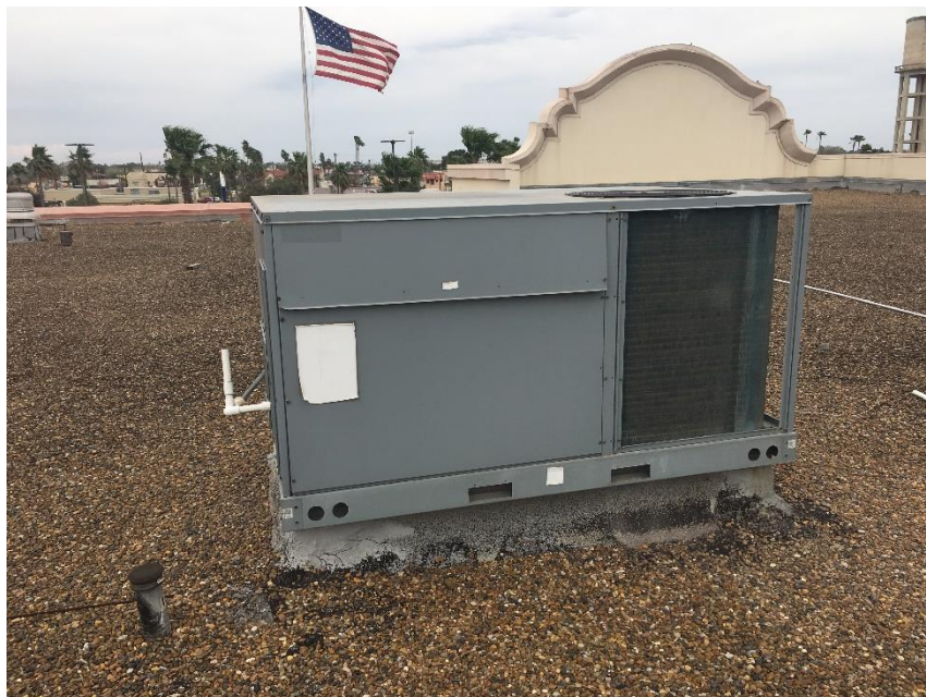
Figure 26: Replaced Roof Top Unit at City Hall
