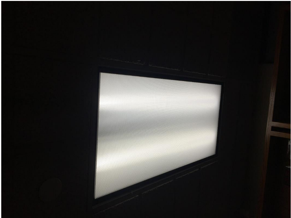
Figure 32: 2x4 LED Light Fixture at Public Library
