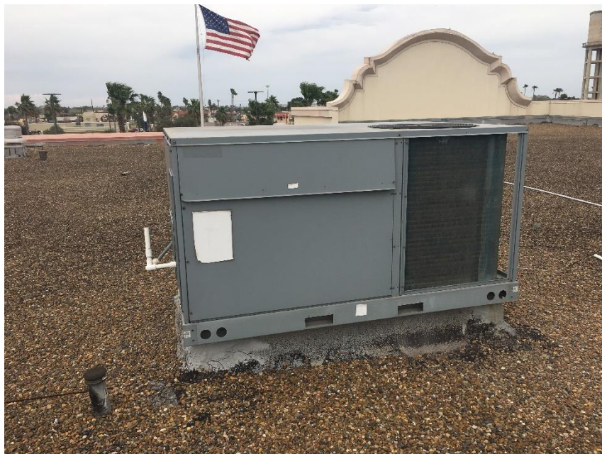
Figure 26: Replaced Roof Top Unit at City Hall
