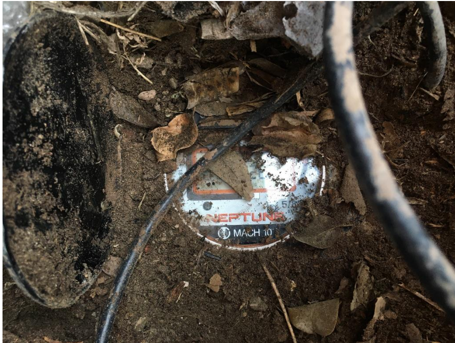
Figure 3: Typical Neptune Mach 10 (meter was covered by dirt and leaves)
