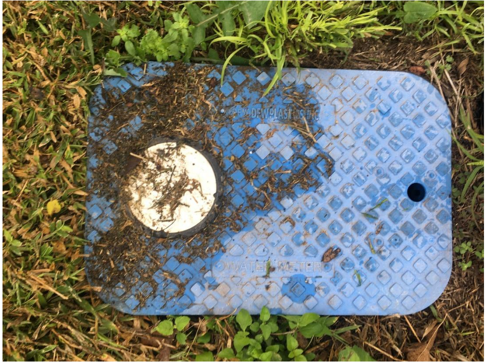
Figure 7: Meter Lid inspected, was properly in-place
