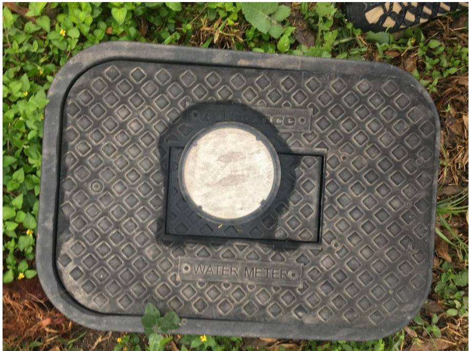
Figure 8: Meter lid was in good condition
