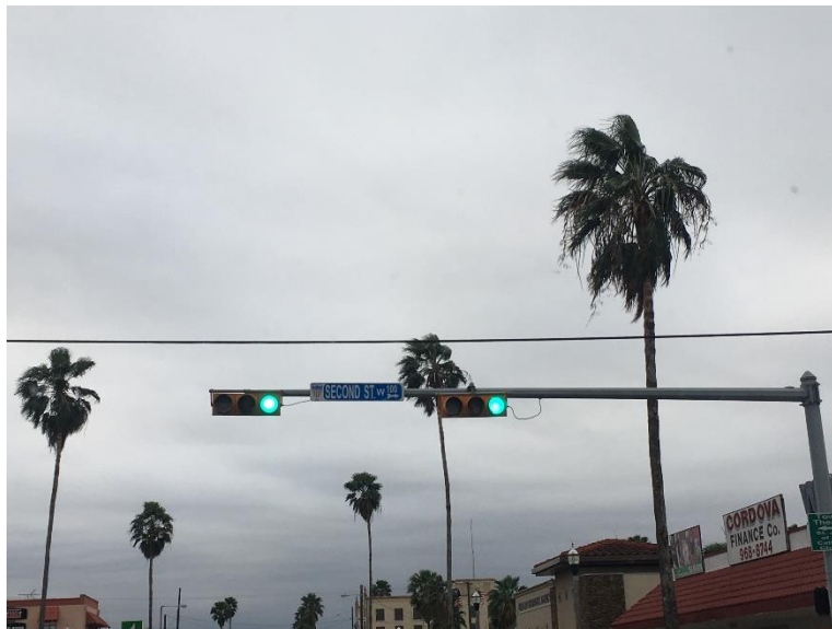
Figure 39: LED Traffic Signal
