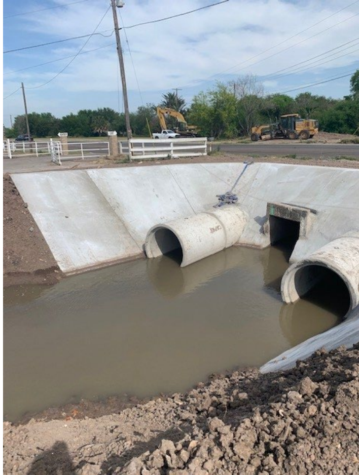
FM 1015 Crossing (West Side)
