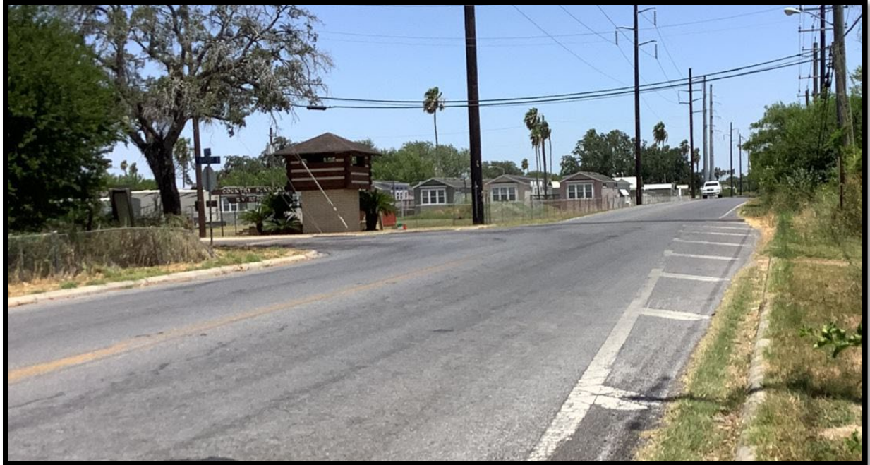
Eastbound approach at 18 th Street
