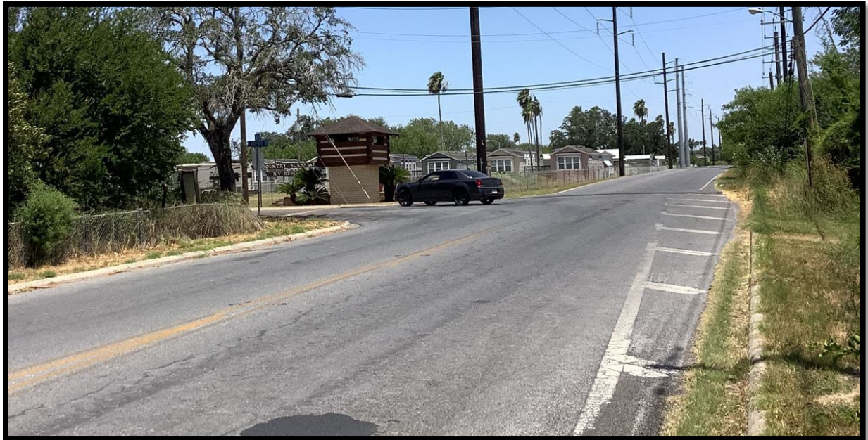
Eastbound approach at 18 th Street
