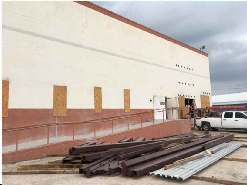
View South elevation. Steel is being staged for installation. Squares above doorway are steel reinforcement for the new door and window openings.
