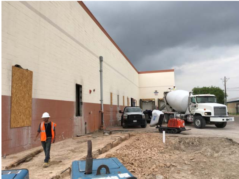
View along the East elevation. Workers are preparing the subgrade for the tower foundation.
