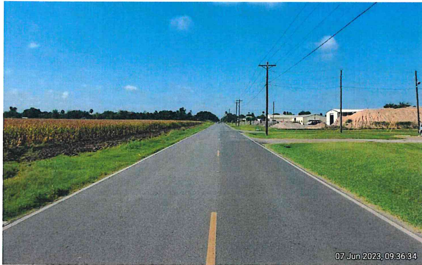
Looking South from the northern property limits on N Mile 6 1/2
