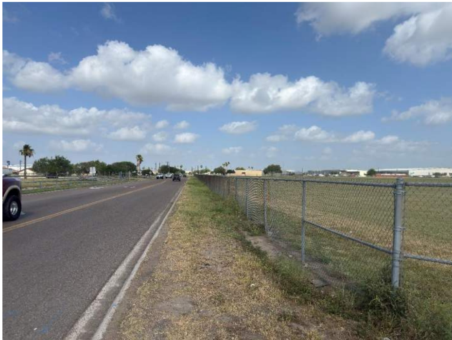
Photo 18: Northwest corner of Vo Tech Dr. and E. Pike Blvd facing West
