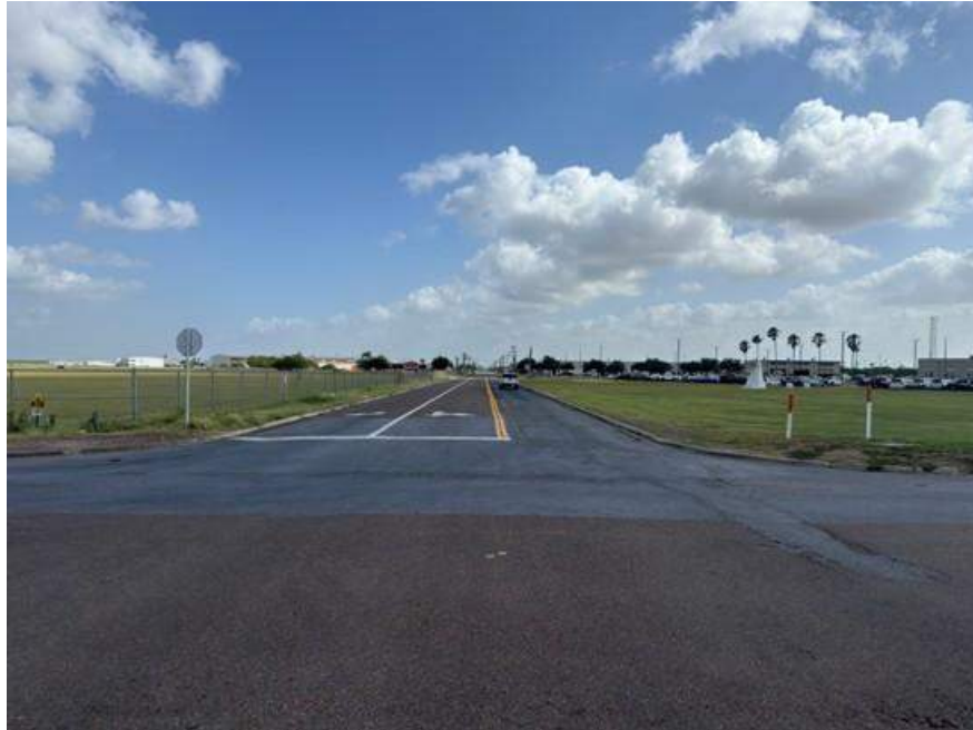
Photo 15: Vo Tech Dr. and E. Pike Blvd facing North
