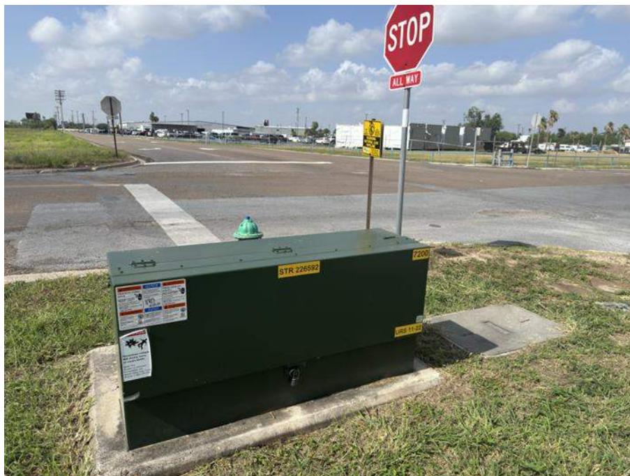
Photo 5: Northeast corner of Vo Tech Dr. and E. Pike Blvd facing Southwest (Presumed transformer, fire hydrant, stop, and warning sign)
