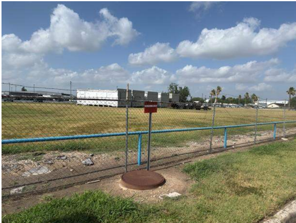
Photo 10: Southwest corner of Vo Tech Dr. and E. Pike Blvd facing Southwest (Warning sign and manhole cover)
