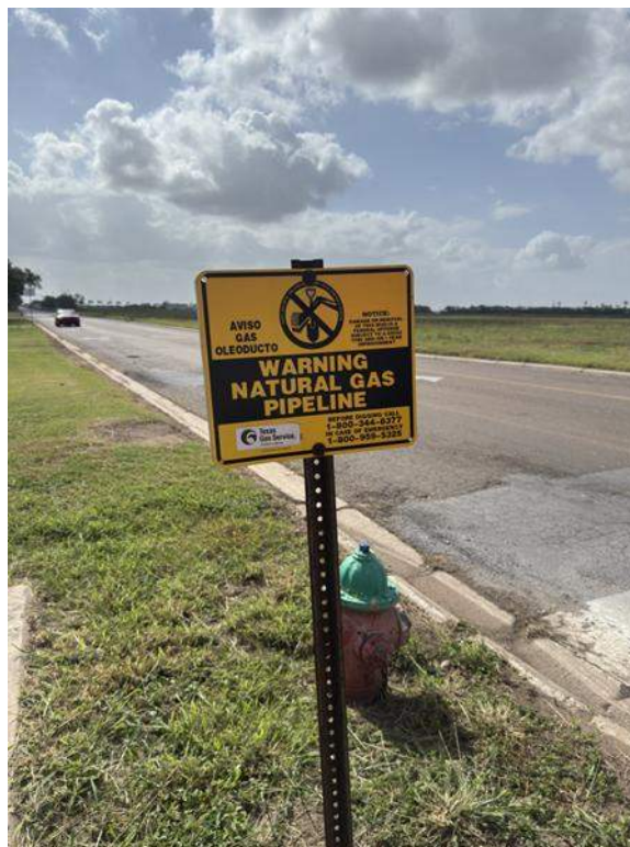
Photo 4: At Northeast corner of Vo Tech Dr. and E. Pike Blvd facing Southeast (Warning sign and fire hydrant)
