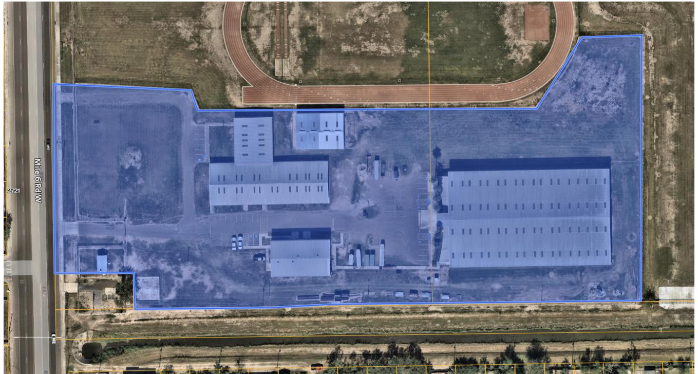
Figure 1. Aerial view of project limits
