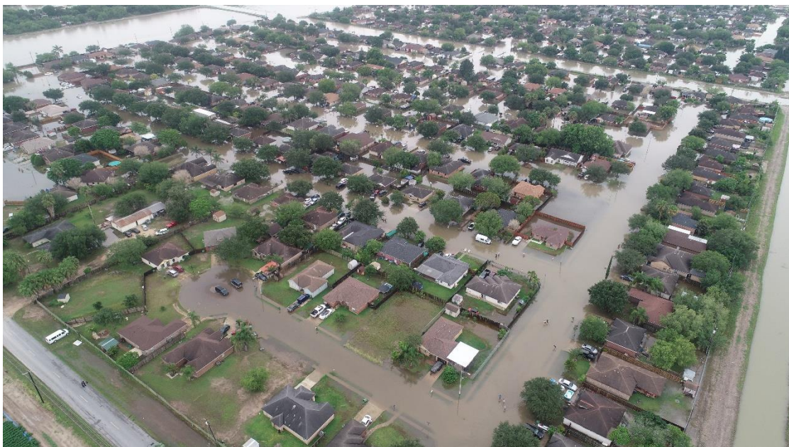
Figure 4. Flood Photo 6/25/2018 at Las Brisas Drive and Mile 9 N
