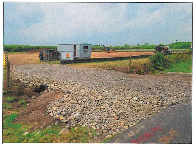
Construction entrance – large stone.
