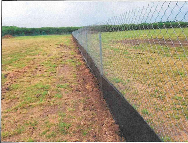
Silt fence in place.
