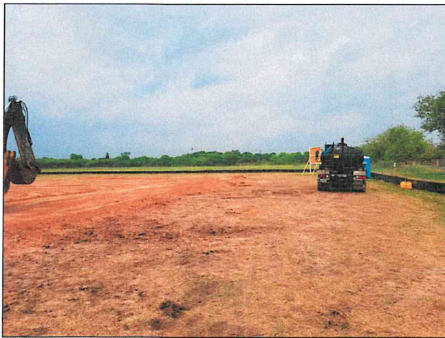
Water truck on site for dust control.
