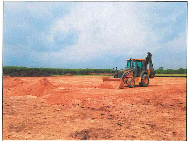
Select fill – 6 inch lifts.
