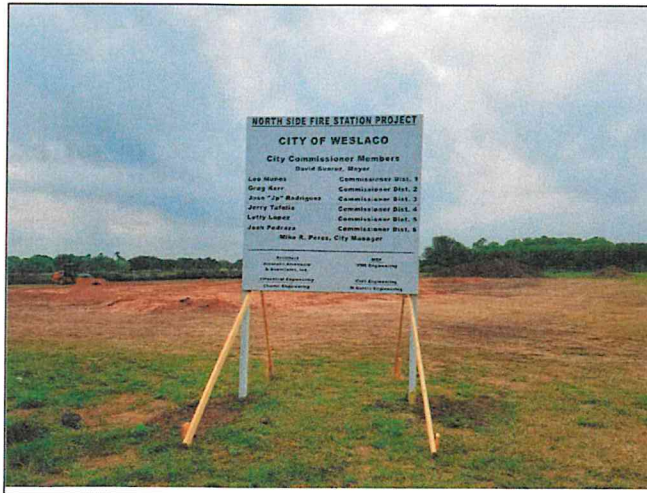
Project Sign is posted on site.
