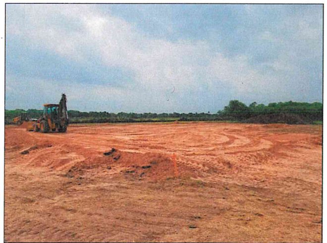
Staking of building corners has taken place.
